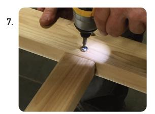
Using a screwdriver or power drill/driver, attach the Rafters to the Posts using the provided bolts through the pre-drilled holes. Once you have attached both bolts on both rafters, flip your assembly over and repeat steps 8 & 9.
