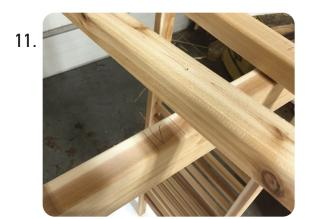
Lay the Purlins on top of the Rafters. There are pre-marked Xs denoting where the Purlins should go on top of the Rafters. Make sure the pre-drilled holes on the Purlins line are also centered on the Rafters
