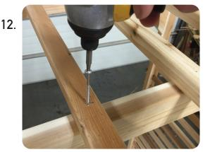
Attach the Purlins to the Rafters using the provided screws through the pre-drilled holes.
