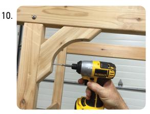
Attach the Bracket to the Post using the provided screws throught the pre-drilled holes. REPEAT STEPS 7 & 8 FOR ALL FOUR RAFTER TO POST CONNECTIONS.
