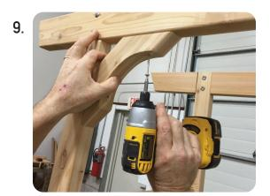
Place the corner Brackets on the inside of the Rafter & Post connection as shown above, making-sure that the flat portions of the Brackets are flush with the flats of the Rafters & Posts. Attach the Bracket to the Rafter using the provided screws through the pre-drilled holes.
